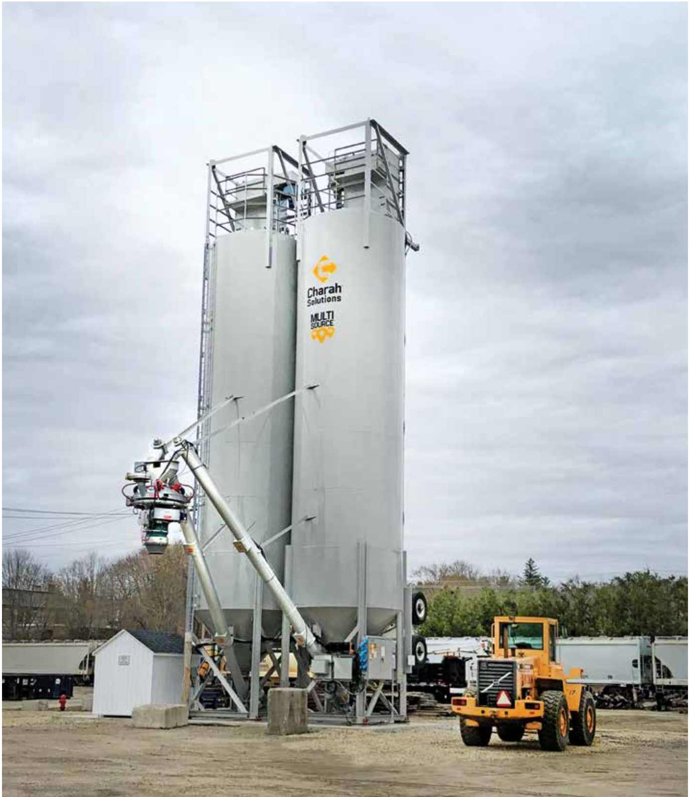
Charah Solutions' Hopedale, Mass., MultiSource® terminal provides concrete product manufacturers in greater New England with access to almost 30,000 tons of quality fly ash.
